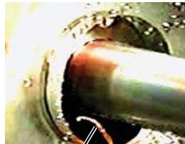
Water Being Pumped into the Bearing Cavity
